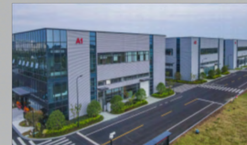
Deli Hangzhou Industrial Park
